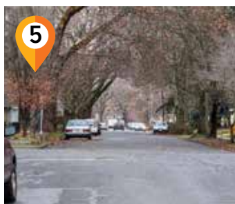
5 Clinton Street - Isaacs to Sumach Replace existing asphalt surface, ADA ramps, water, sewer
