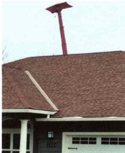
See Above: View from front yard of 1135 Chestnut Drive.
