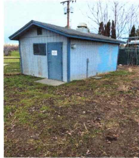
See Above: This is the equipment building for the cell tower with graffiti painted on it. This cell tower and its equipment are not in keeping with the neighborhood and will be clearly visible.
