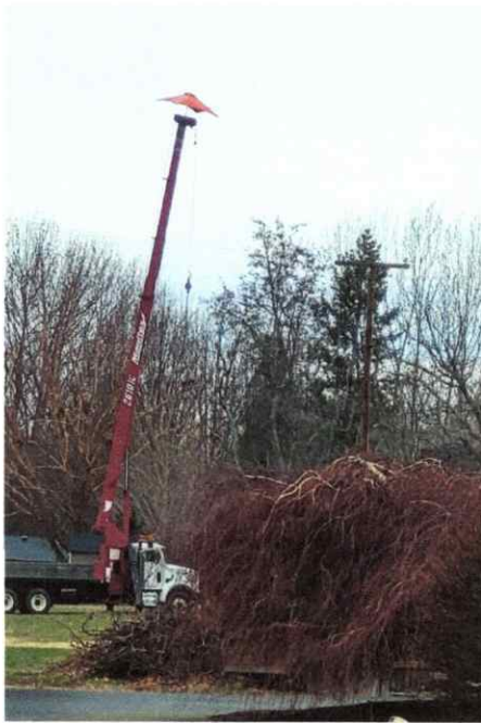
See Above: View from back parking lot of church. The 30' high power lines would be 20' from the cell tower. The cell tower would be 35' higher than the power poles.
