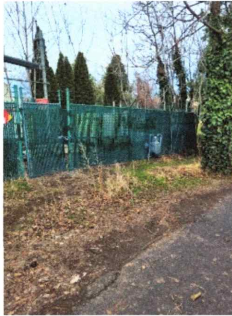
See Above: Unsightly view of the fence around the base of cell tower at Municipal Golf Course. The trees are voluntary sucker trees. No one maintains the aesthetics of the base of the cell tower.
