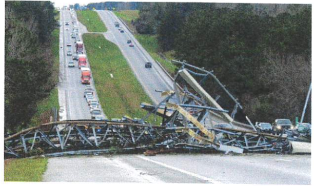
Cell tower felled by tornado across U.S. Route 280. Smiths Station, Lee County, AL, March 3, 2019 https://www.nytimes.com/2019/03/03/us/tornado-alabama-georgia-deaths.html Photo credit: Mike Haskey/Ledger-Enquirer, via Associated Press
