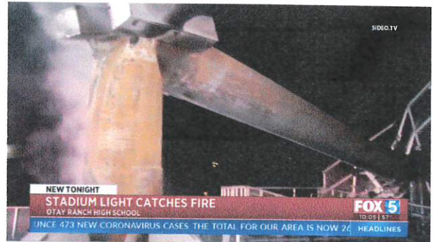
A light pole holding cellular antennas at Otay Ranch High School caught fire, damaging the stadium Chula Vista, CA, March 9, 2021 https://fox5sandiego.com/news/local-news/stadium-light-catches-fire-at-south-bay-high-school/ Source: fox5sandiego.com
