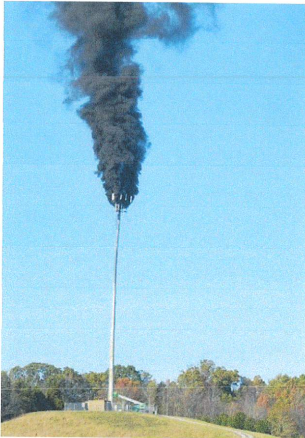
Cell tower fire caused by improper welding. Greenville, TN, Nov 4, 2014 https://www.greenvillesun.com/xml/nitf/flames-damage-verizon-wireless-tower/article_1619f00e-5383-
