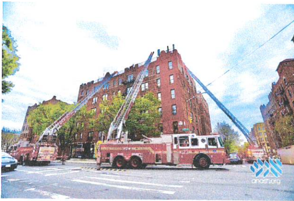
Electrical malfunction causes fire with rooftop cellular antennas Brooklyn, NY, April 18, 2021 https://ehtrust.org/firecell-tower-brooklyn-new-york/ https://anash.org/fire-extinguished-on-roof-of-crown-heights-apartment-building/ Photo credit: Berel Meyers/Anash.org
