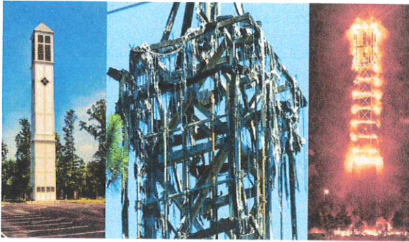
Cell tower fire (in a church steeple) caused by electrical/mechanical issues. Hanover, VA, June 26, 2020 https://www.nbc12.com/2020/06/26/cell-phone-tower-hanover-catches-fire/ Source: Hanover Fire and EMS
