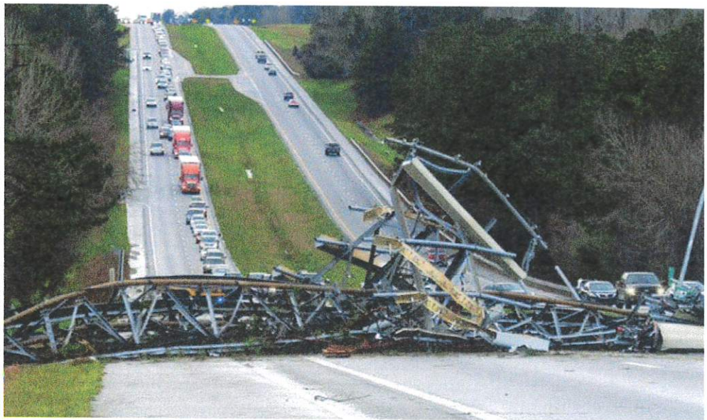
A fallen cell tower lies across U.S. Route 280 after tornadoes touched down in Alabama, Georgia and Florida. Smiths Station, Lee County, AL, March 3, 2019
