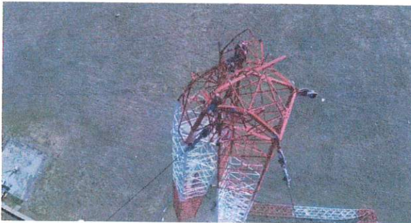
Tornado damages tower array Moore, OK, March 25, 2015 http://qrznow.com/tornado-damage-to-legendary-koma-
