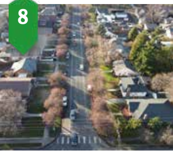
8. Chestnut - 2nd to Howard IRRP Water, sewer, roadway Summer 2023-Summer 2024
