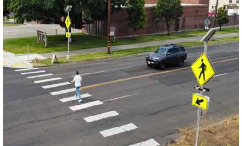
Installing a rectangular rapid flashing beacon (RRFB) is an effective way to improve safety for pedestrians crossing the road at congested or potentially dangerous intersections
