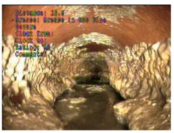
This photo of the inside of a sewer pipe in Walla Walla shows what FOG buildup looks like. FOG reduces the diameter of the sewer pipe and can create blockages.
