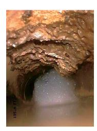
This is the Inside of a sewer line with soap bubbles floating on the wastewater and FOG hanging from the ceiling of the pipe. The diameter of the sewer pipe is reduced, creating a potential site for a blockage.
