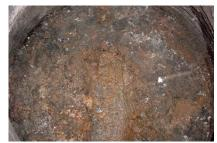
Looking down from the street, this is the view of the bottom of a sewer manhole that has a solid layer of FOG buildup.
