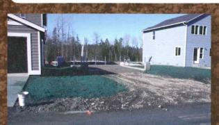
The next step is to place rock pads for roads and driveways. Once foundations are in and houses are framed and sided, 14 inches of compost-amended reused soil is placed (to allow for settling to 12-inch finish grade). The compost blend prevents erosion, so work can proceed year-round.
