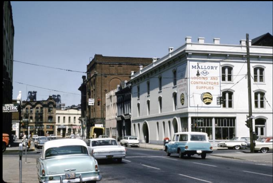
United Carriage Building, Portland, OR
