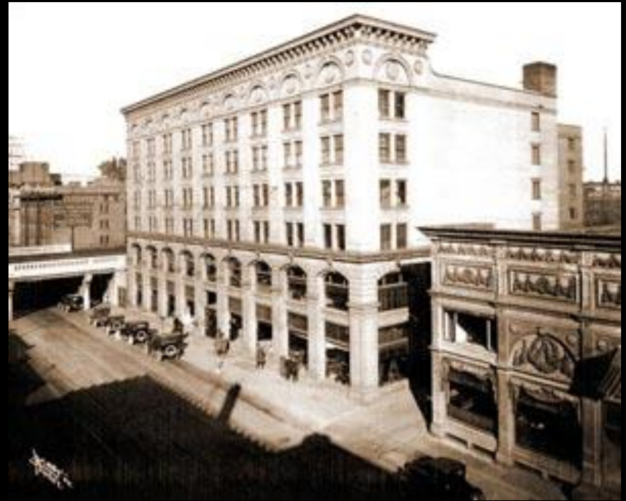
Holley Mason Building, Spokane
