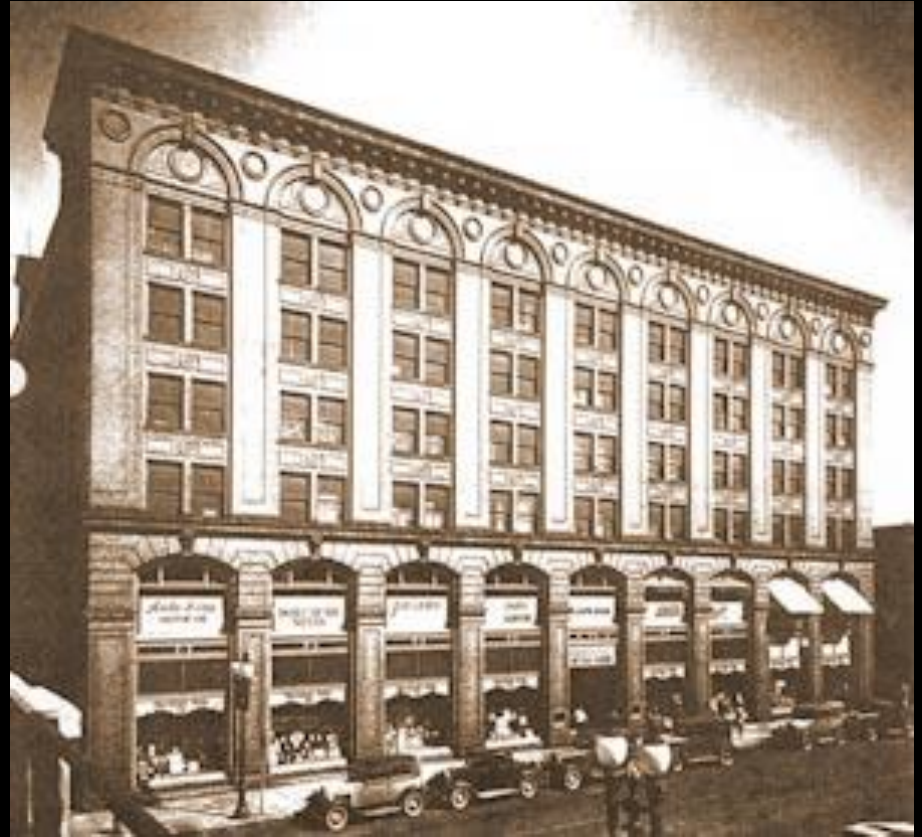
Holley Mason Building, Spokane
