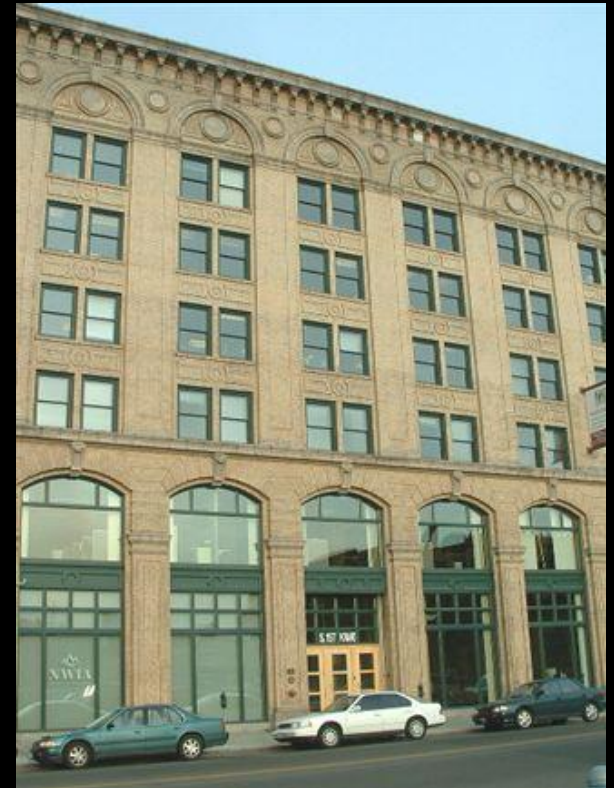
Holley Mason Building, Spokane
