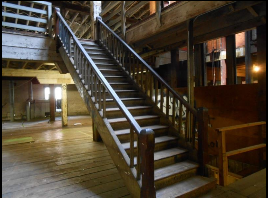
United Carriage Building, Portland OR
