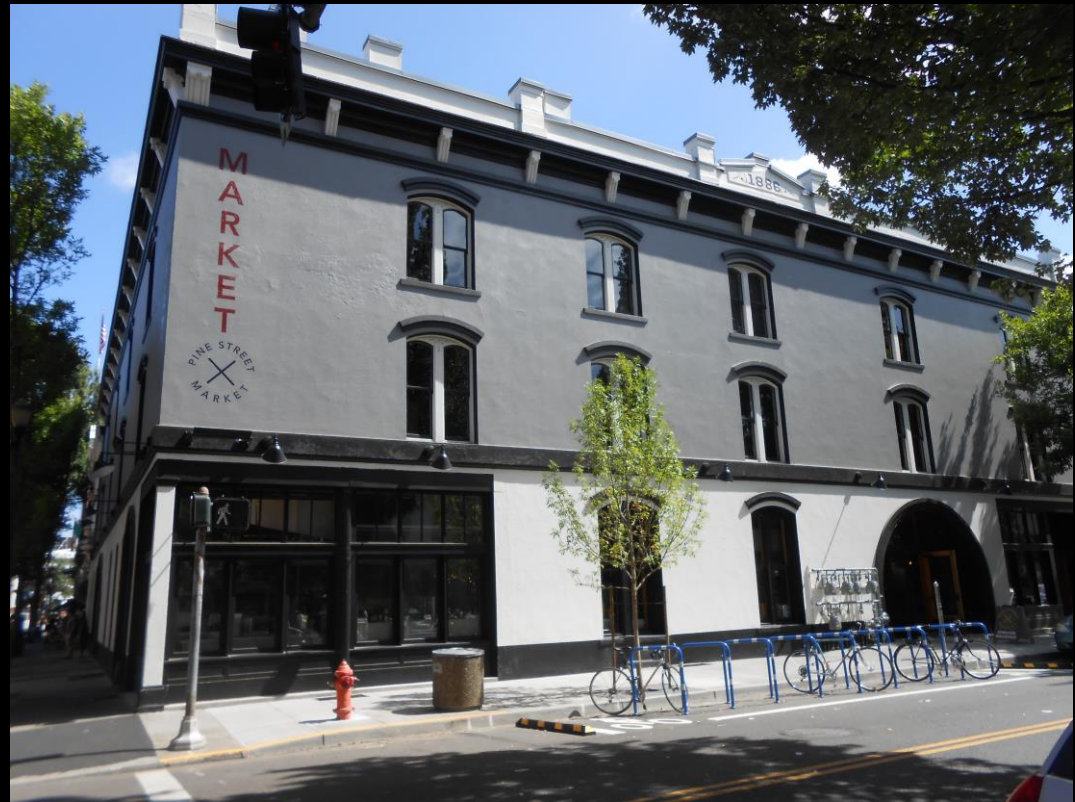
Pine Street Market (United Carriage and Baggage Transfer Company Building) Skidmore/Old Town National Historic District, Portland, OR
