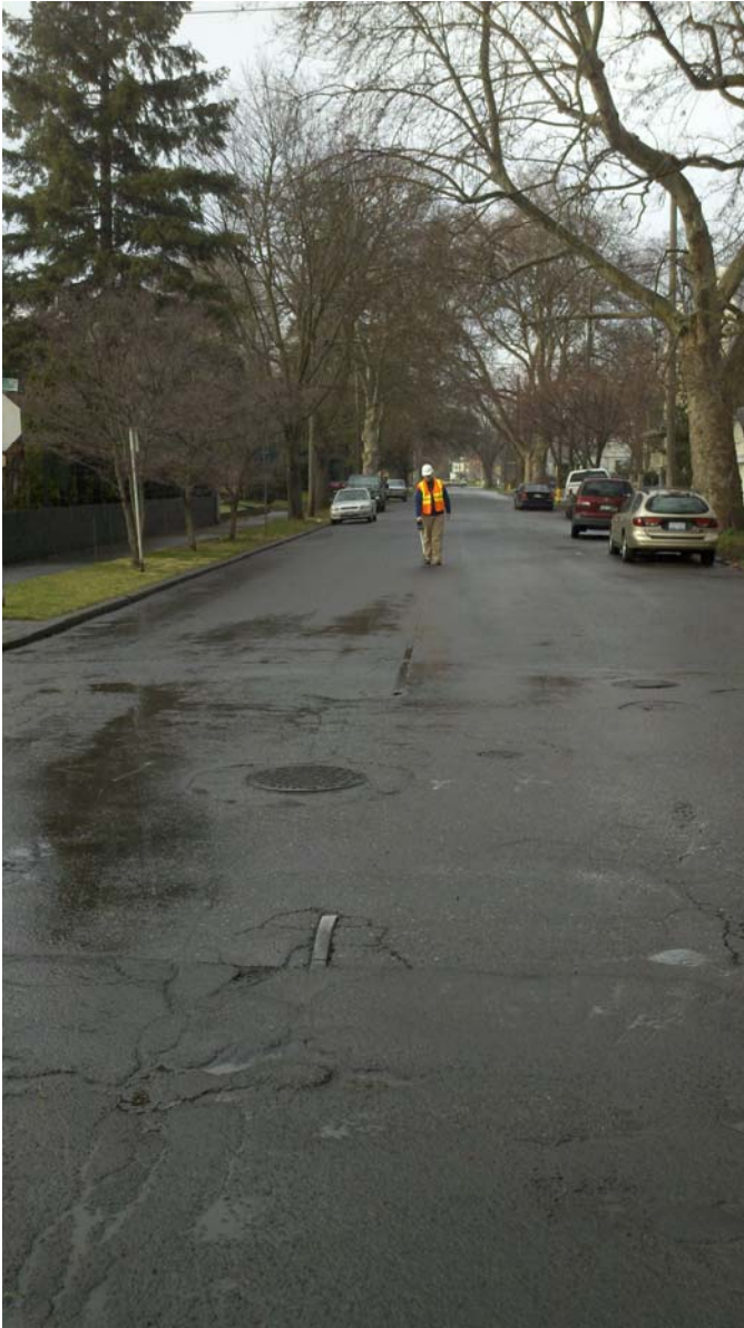
Fig. 11 Facing North on Clinton Street, through the intersection with Boyer Avenue, Exposed track in foreground.
