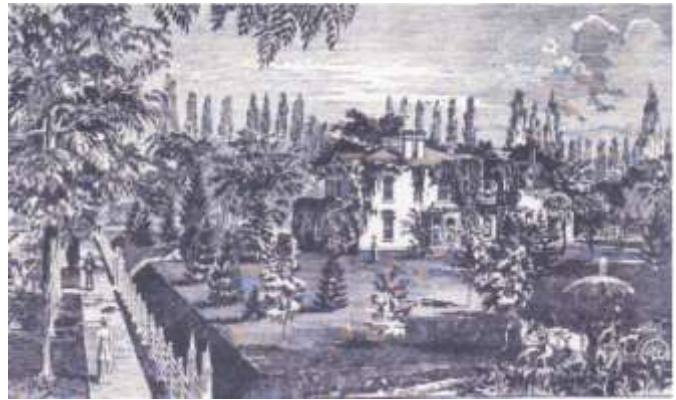
Figure 1. Walla Walla house featured in the October 1889 issue of The Northwest Magazine.
