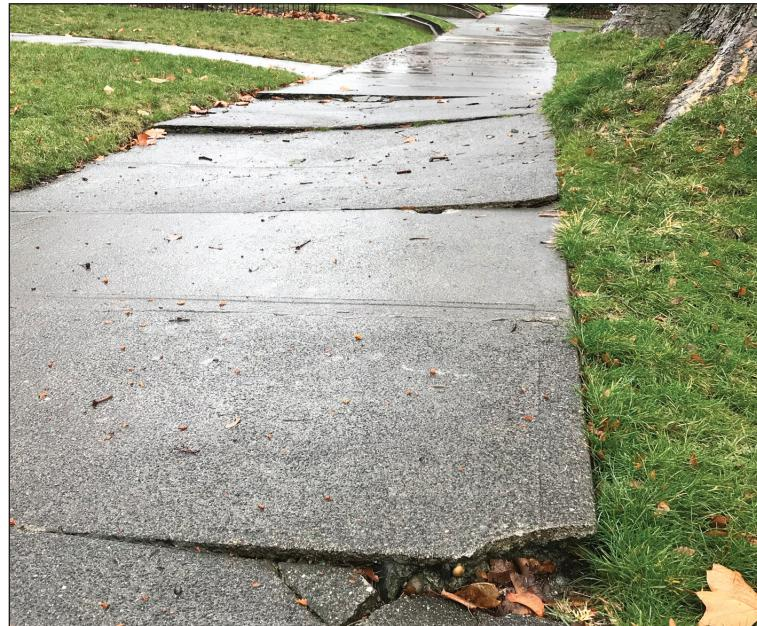
of problems. The roots of some mature trees in planting strips are pushing up sections of sidewalk, creating tripping hazards.
