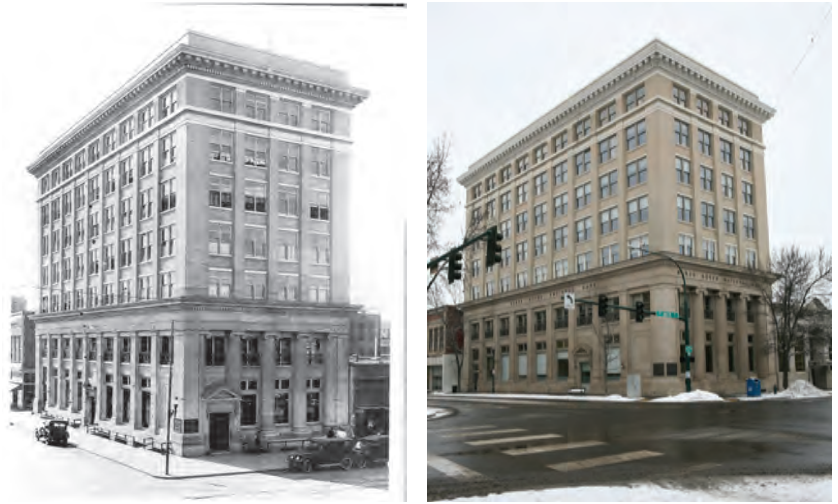
Ca. 1910 view of the Baker Boyer Bank (left) and a 2017 view of the bank. Historic image courtesy Whitman College and Northwest Archives. Contemporary image courtesy Artifacts Consulting.
