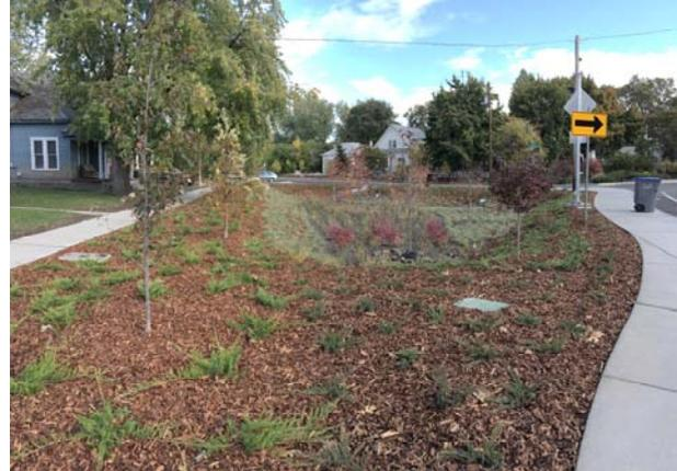
sidewalk and other available landscape areas. Subsurface infiltration galleries will be used to retain higher flows allowing runoff events to naturally infiltrate for groundwater recharge. This approach avoids large concentrated flows to surface waters, which often contain high levels of pollutants and minimizes the negative effects of urbanization on the environment.
